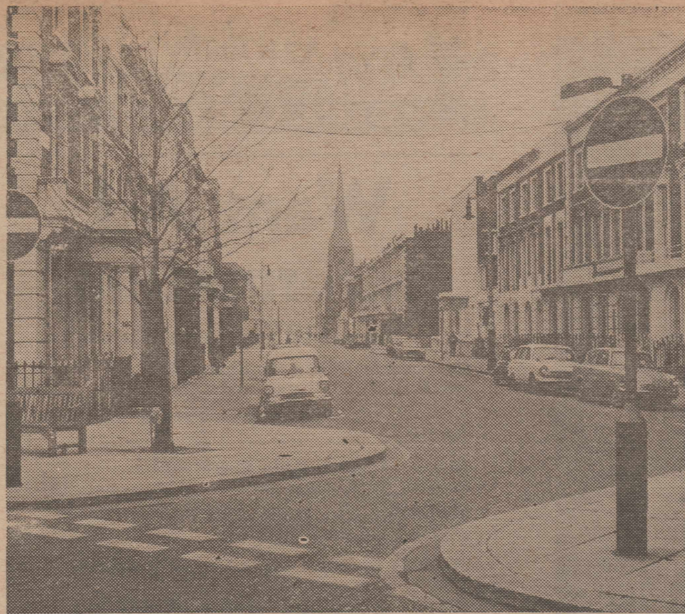
LONDON'S ANSWER to speedsters swerving and careening through quiet neighborhood streets. Wide streets give way to very narrow bends at each corner. Speeders soon tire of accelerating when they have to apply brakes quickly to make turns.
