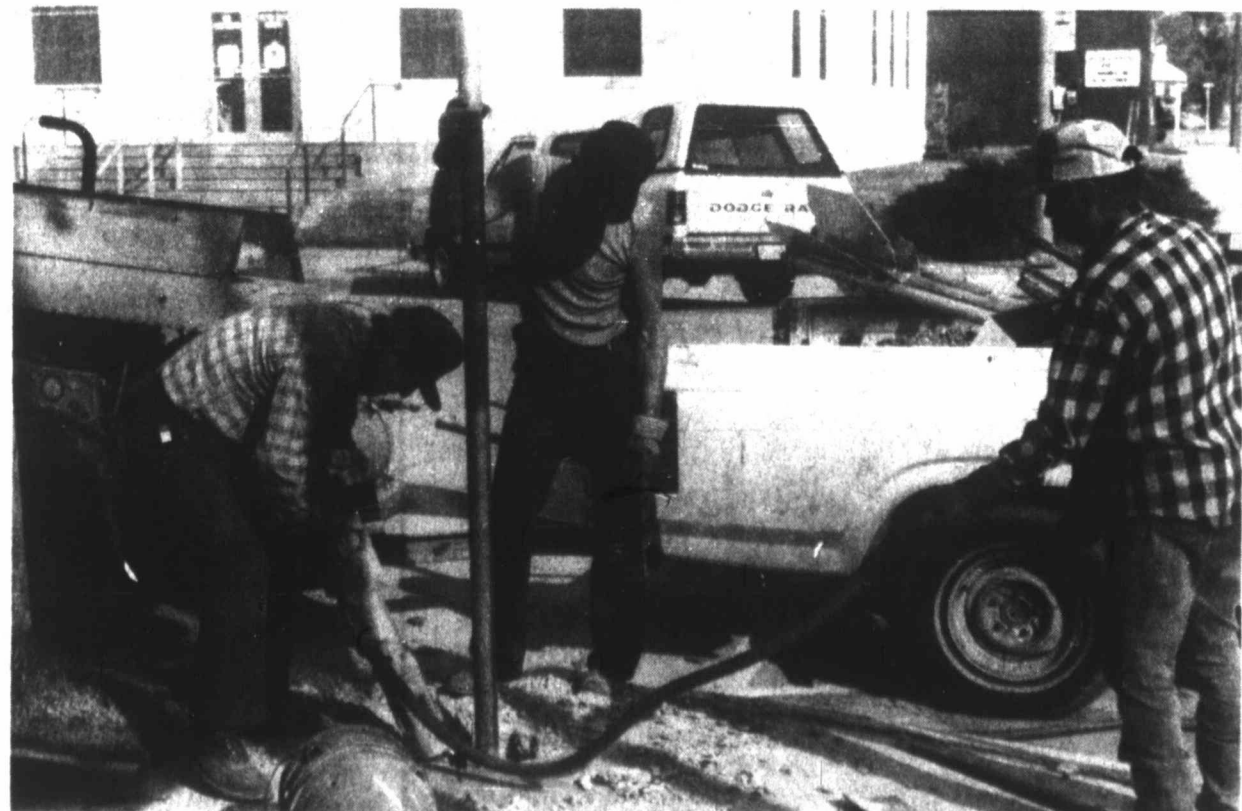
PUTTING UP SIGNS - These city workers were busy Tuesday erecting four-way stopsigns at the intersection of Third and Walnut streets. The 4-way stopsigns will replace the lighted signal at that intersection.
