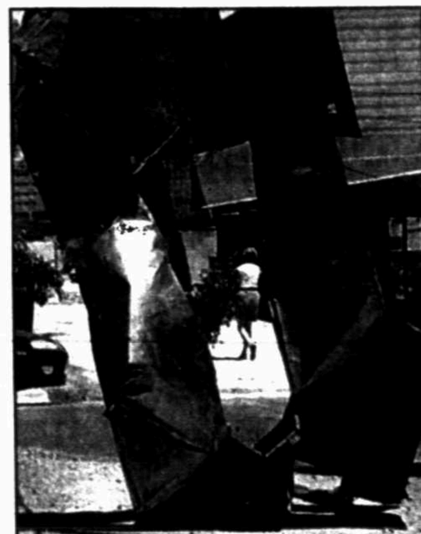
Billie Lanier, carrying tree branches to a trash bin Sunday afternoon, is framed by copper roofing that the Saturday night winds peeled from a building near the intersection of G and Wall streets.
