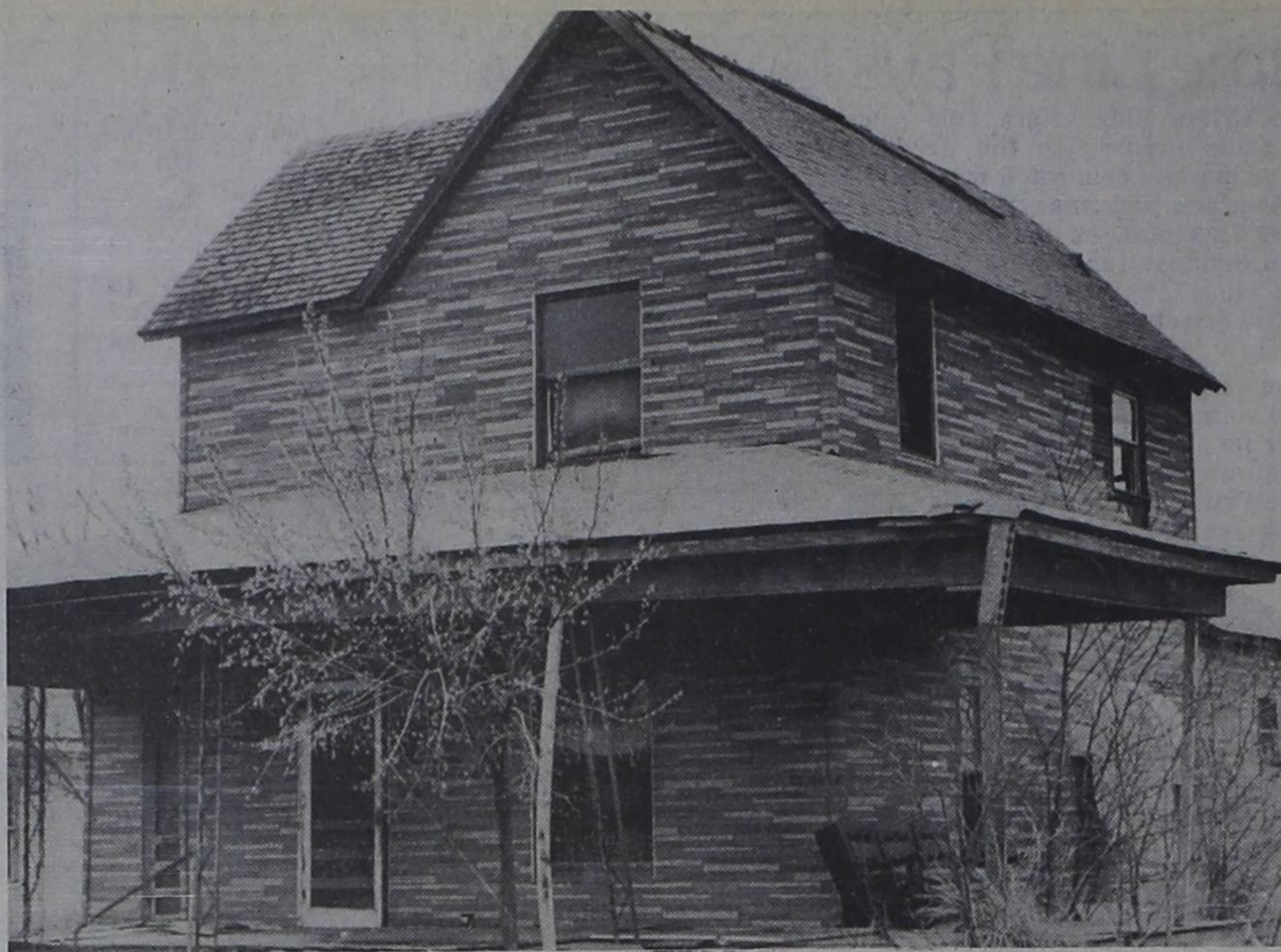
This house on West 11th St. is the subject of condemnation proceedings by the city council. (see story on Page 1)(Photo by Tim Burnett)
