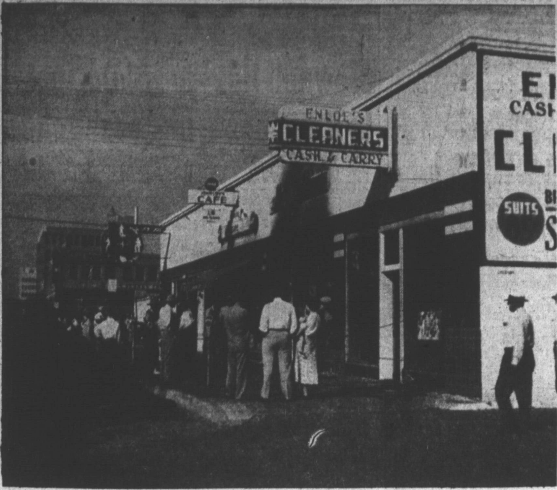
AFTERMATH — Interested Pampans this morning gathered around the fire lines set up in a half-block area on East Kingsmill, gutted early today by Pampa's worst fire in six years. Johnson's Cafe, Melody Manor and Enloe's Cleaners, in the foreground of the picture, were total losses. The Sportsman's Store and H. W. Waters Insurance Agency, toward the background, had extensive damages but were still usable. In the foreground, right, can be seen a board of cartoons, one of the few things in Enloe's not hit badly by the fire. Estimated damages are $100,000 to all five concerns, according to Fire Chief Ernest Winborne. (News Photo)
