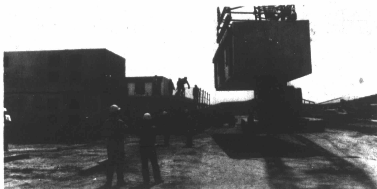
UP, UP AND AWAY: The last of 144 precast cell modules was lifted into place Friday afternoon at the Wallace Unit by employees of the H.B. Zachary Company of San Antonio. Each module this size weighed in at 120,000 pounds and the crane doing the lifting is capable of lifting about four of these at one time. It took 14 trucks to bring the crane in pieces from Florida.
