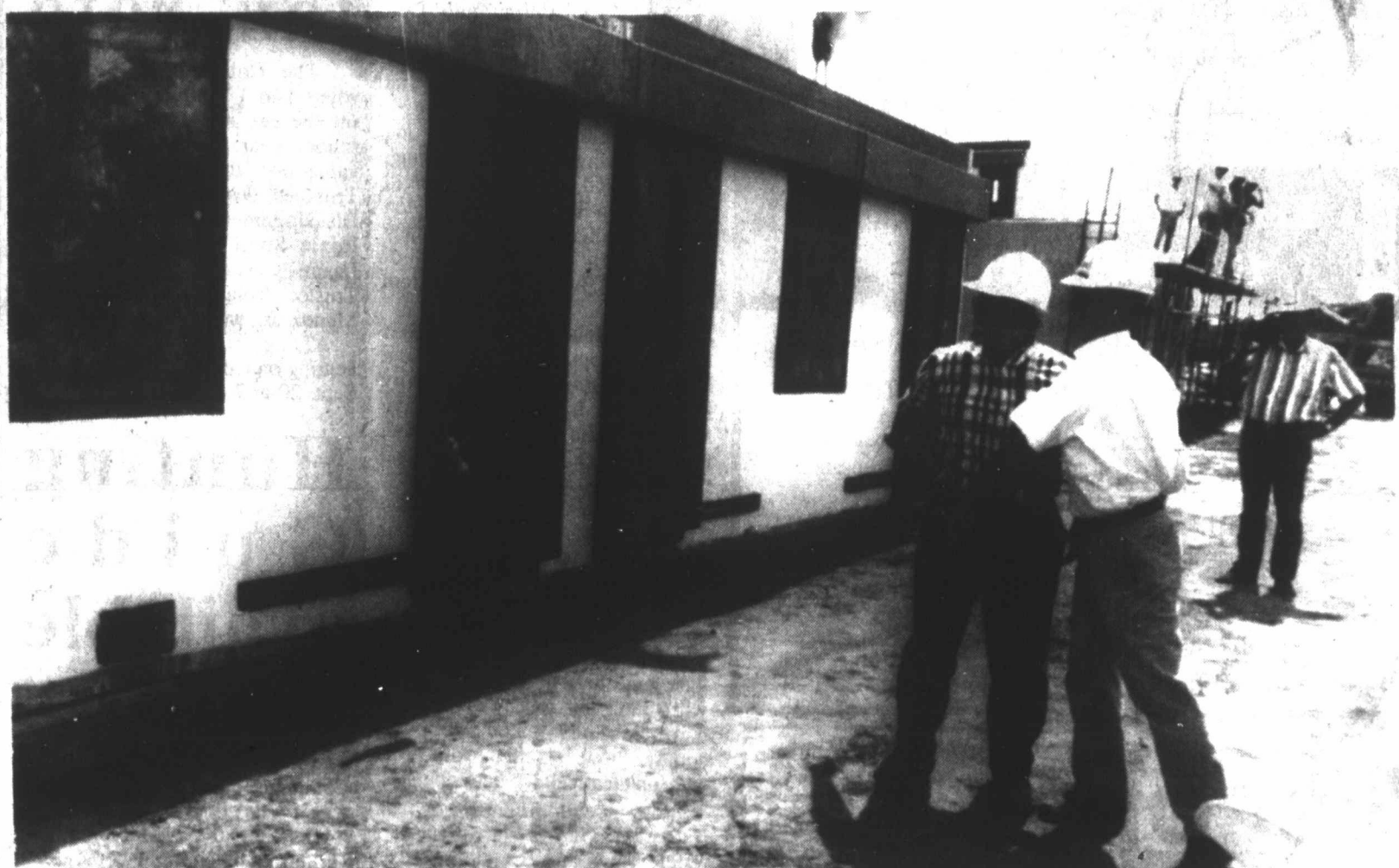
THE LAST ONE: Frank Toland, Texas Department of Criminal Justice Construction Coordinator (on the left) and Bill Harbert Construction Company vice president, Howard Dyer-Smith, look over the last of 144 pre-cast
