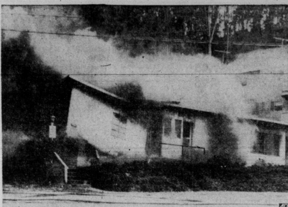
APARTMENT HOUSE FALLS INTO HOLE—This burning 10-unit apartment house that was constructed atop a large railroad tunnel in San Rafael, Calif., is seen falling into a gaping hole made when the tunnel collapsed as a fire burned out its wooden supports. The apartment building was evacuated before it collapsed, however one fireman was killed when the tunnel caved in. (AP Wirephoto)
