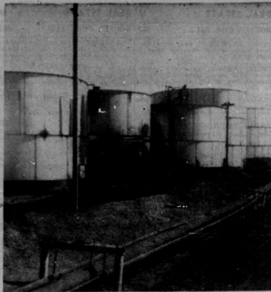
AFTER UNLOADING the raw material is stored in these storage tanks. Storage capacity is 49,000 barrels. Processing capacity is 450 barrels per day.
