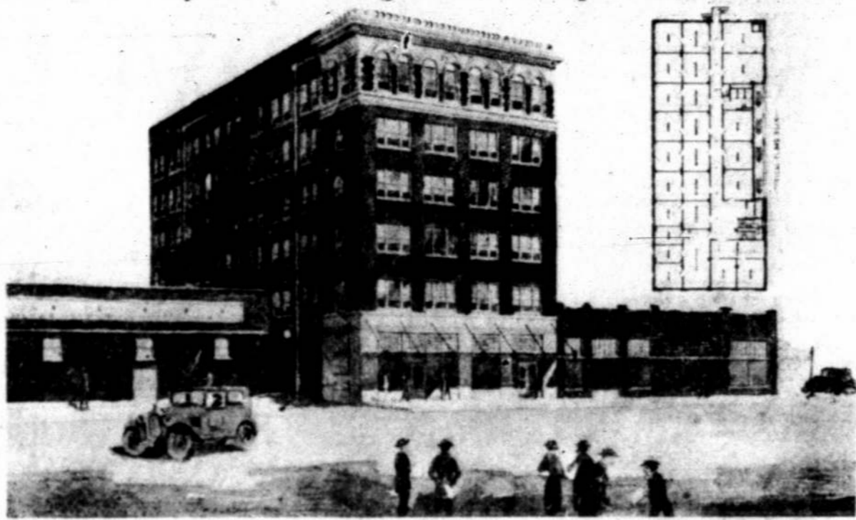
The six story Myrick building now being erected on Avenue J, and nearing completion, will not only be one of the largest office buildings on the South Plains but one of the most modern. It is a unit of the million dollar construction program which has been going on in Lubbock since the first of the year, and which during the first two weeks of July has been augmented by a steady building of residences, amounting to more than $100,000.
