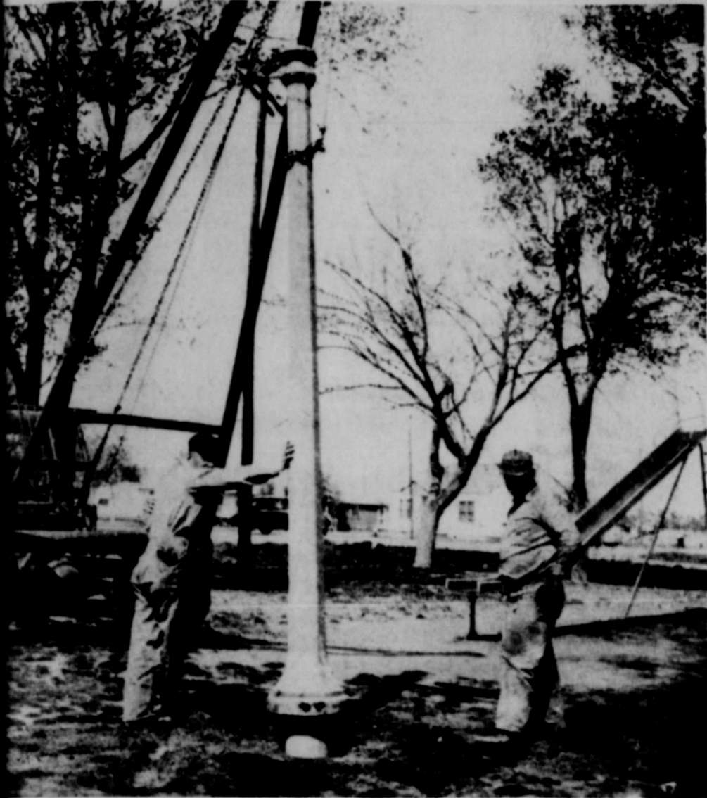
WORK LIGHTS —Jess Porter and Leon Morgan, city employees, are shown with one of the four projected this week at the city park to provide light during summer activities near the play park. This is one of the many improvements being made at the city park this year.
