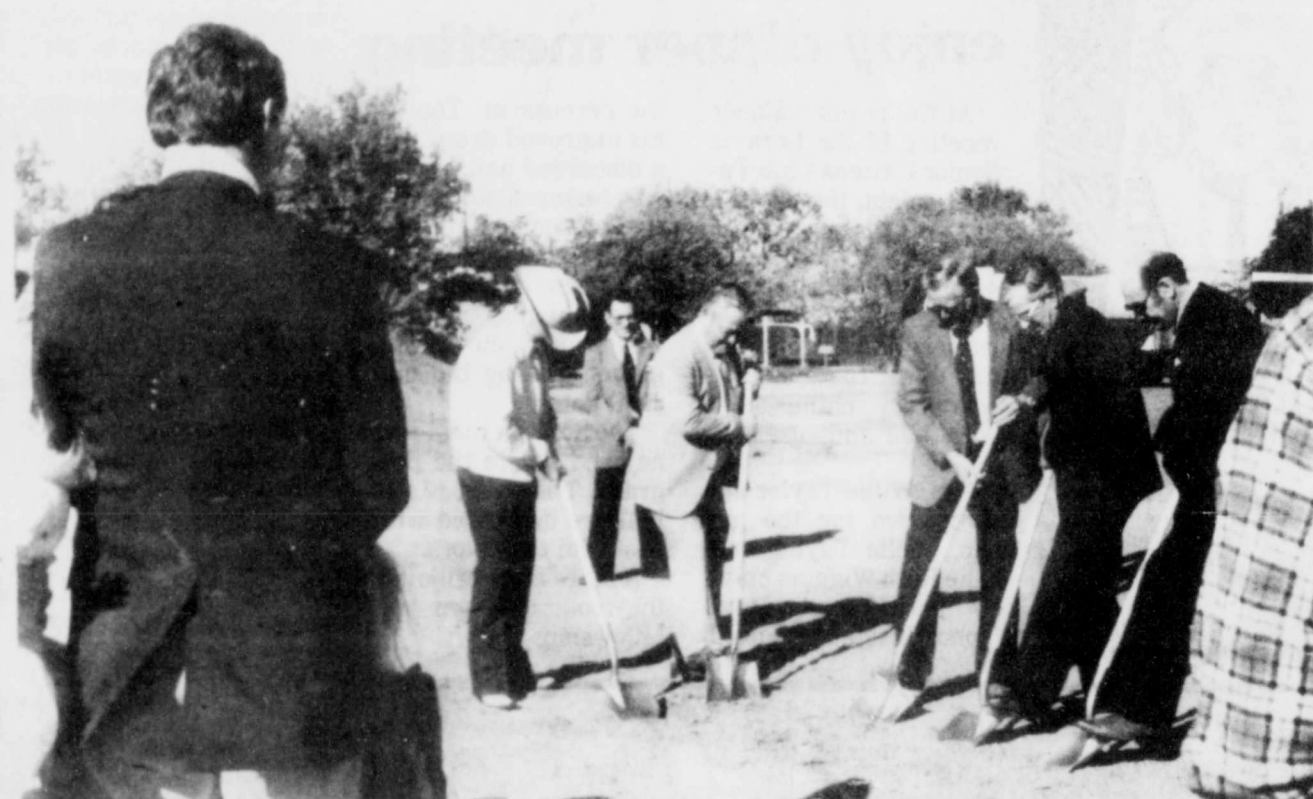
THE BOARD OF DIRECTORS at First Western Savings & Loan Association broke ground on their new $1,000,000 building Monday morning. Turning the first shovel of dirt are (left to right) Buddy Hertenburger, B. B. Hardee, Glen Hemphill, Jack Hollis and Charles Root.
