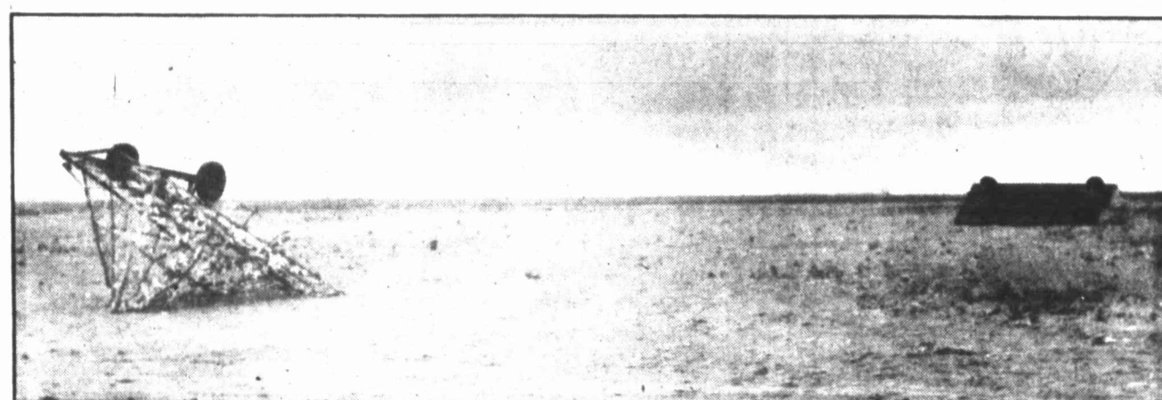
Tornado-force winds wrought extensive damage, top photo, on the Flowergrove Co-op gin west of Ackerly Tuesday night. The scattered remains of cotton trailers, below, dotted the land around the Co-op.
