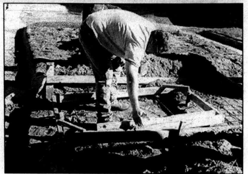
DANNY MARTIN, project manager for the Texas Department of Transportation's Colorado City street project, checks the slope of one of the wheelchair ramps being installed along a stretch of Chestnut Street. Construction crews are currently filling the frames with cement.
