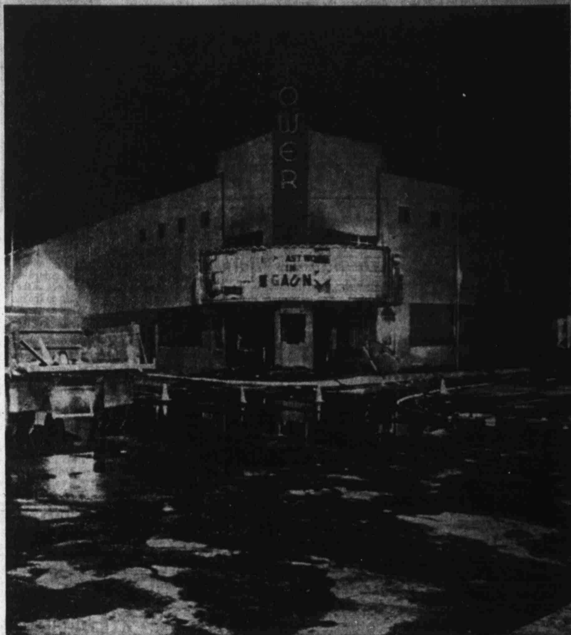
THEATER'S SHELL — Guttered remains of the Tower Theater stand in mute testimony to the fury of an afternoon fire that raced through a major downtown area of Portales Friday. (Staff Photo by Milton Adams)
