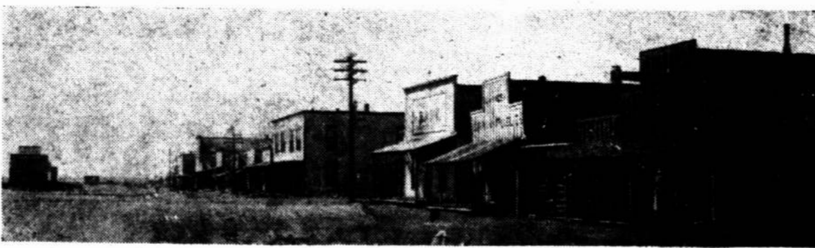
In the foreground of the above scene, looking southward along Austin Street, is the Lamesa hotel, owned and operated by Mr. and Mrs. Jarvis Stockton, which stood where the Dawson County Abstract now is; the general merchandise store operated by J. M. Baker and J. E. Garrison; the Dawson County Bank (now the First National); the Lindsey building which housed the J. J. and M. C. Lindsey abstract office and the E. Y. Lindsey drug store; W. B. Looney barber shop, a grocery store; R. L. Meek Cafe; J. J. Curlee dry good store; First State Bank (now Lamesa National); W. R. Kelley hotel and in the distance (left) the J. E. O'Quin drug store.
