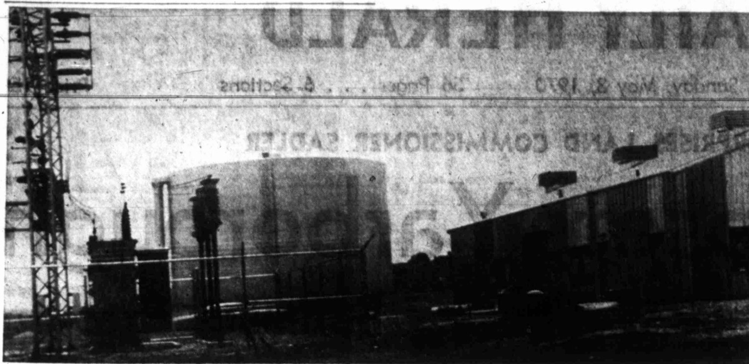
ONE OF SIX NEW PUMP STATIONS BUILT IN WATER DISTRICT EXPANSION Spade Ranch station has million-gallons storage, 17,000,000 GPD rating
