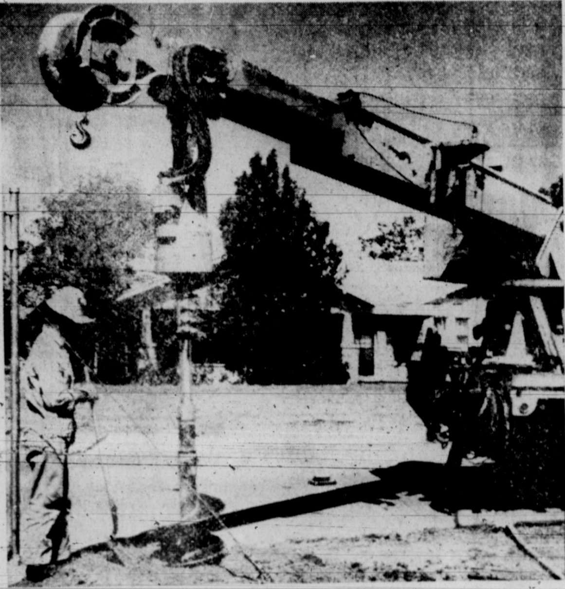
Street Lamp Installation
