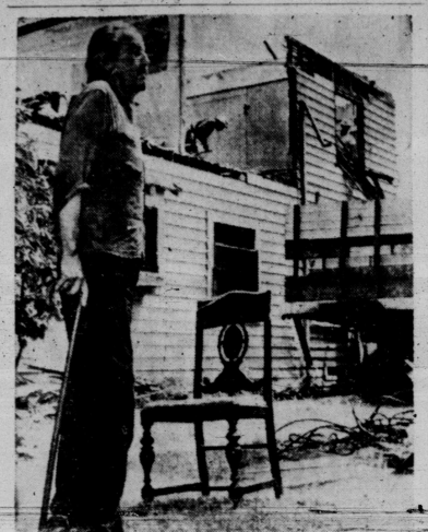
REFUSES TO LEAVE OLD HOME —Arthur F. Hansen, 56, stands near the building that has been his home since 1926, in Los Angeles, as a wrecking crew tears it down to make way for an apartment house. The old house has been sold by a relative of Hansen's who owned it. Hansen, who says he is retired and without money, has been living in the lower floors while upper floors were demolished. Later he was arrested for occupying a house condemned as unsafe. (AP Wirephoto)
