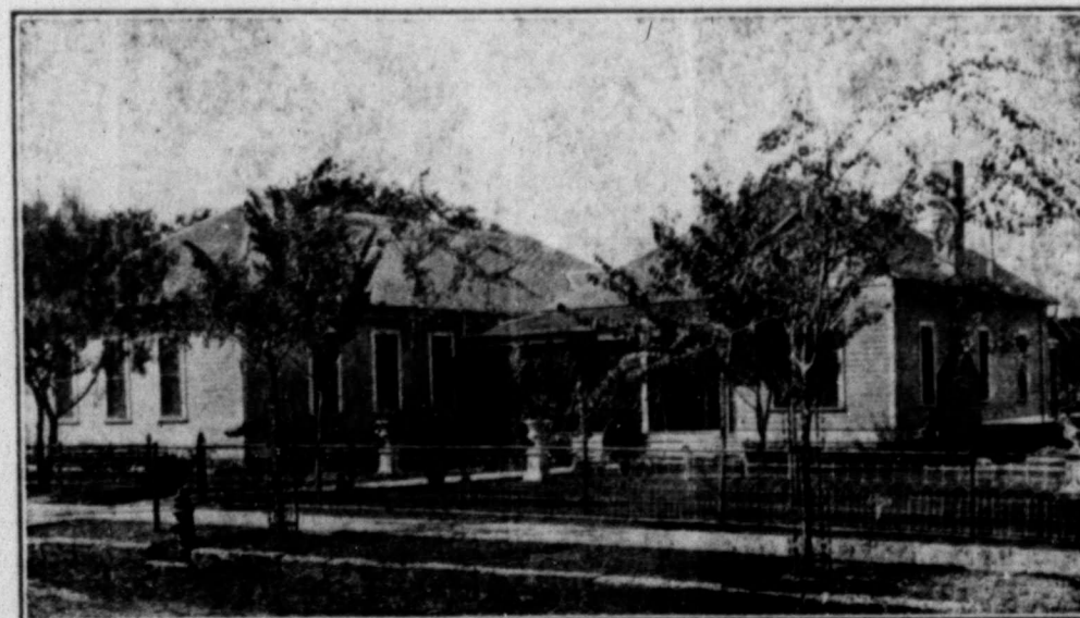
St. Mary's Convent. Besides housing the faculty it accommodates young lady boarders.
