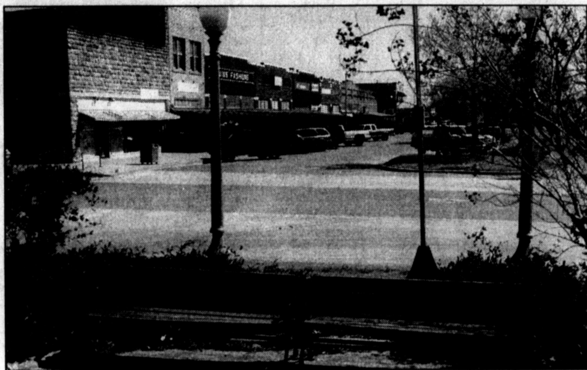
DOWN ON MAIN STREET in Post, Texas are a group of storefronts that have been renovated and refurbished as part of the Main Street Program. Post has participated in the program since 1987 and has attracted tourists because of its historic downtown.
