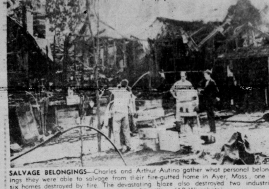
SALVAGE BELONGINGS — Charles and Arthur Autino gather what personal belongings they were able to salvage from their fire-riddled home in Ayer, Mass., one of six homes destroyed by fire. The devastating blaze also destroyed two industrial plants and the damage was estimated at $4 million. (AP Wirephoto)
