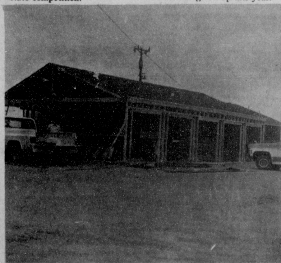
VIOLA'S UNDERGOING FACELIFT, ENLARGEMENT -Viola's, a popular Mexican-food restaurant in west Muleshoe is currently undergoing a facelift. Viola Anzaldúa said the seating area is being enlarged to accommodate 80 diners, along with a new kitchen area, new restrooms, new carpet and decorations. Arches will be constructed across the front of the restaurant and in the near future, Viola's will be featuring an all-new look, but serving the same good food.
