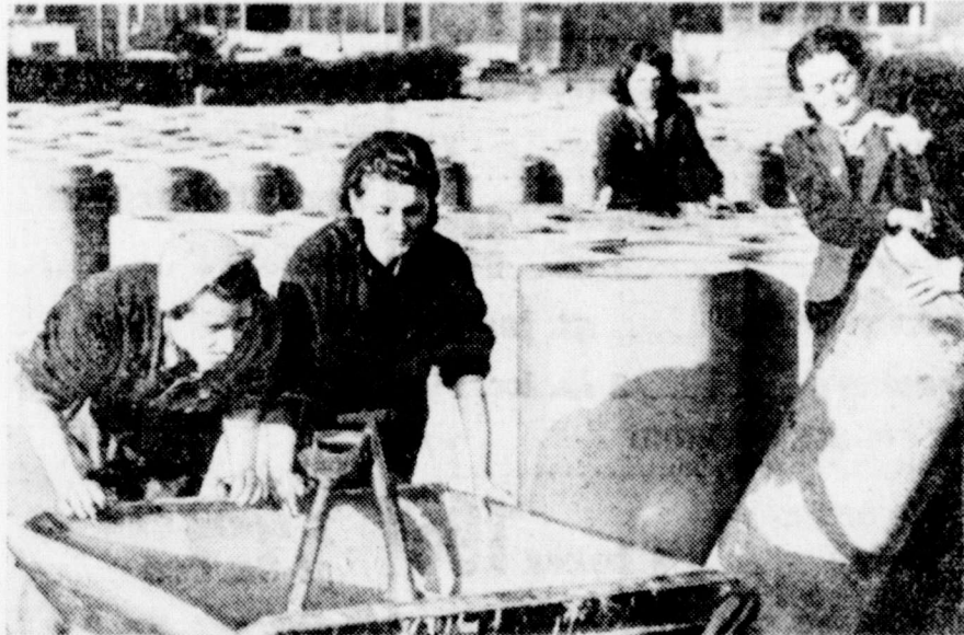
WHEELING IN THE CONCRETE.
