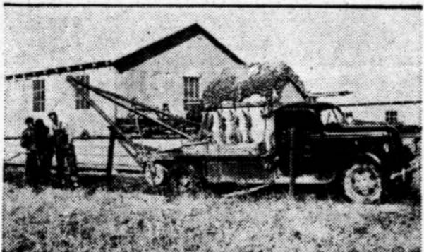
Construction Cruiser on Wheels carrying everything required for construction for a field—from a pair of pliers to a pole-holing winch, a self-sufficient workshop for a crew of six. Bing Barron, Big Spring, Wayne Gregston, Midland, and Doug Rayburn, Big Spring, are the men shown working on a which line.
