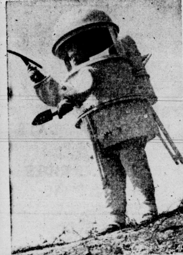
"MOON WORK SUIT"—A man peers from inside of what is described as an experimental two-piece lunar exploration suit. The suit was developed by the Republic Aviation Corporation of Farmingdale, N. Y., which says it is meant to be "working clothes" for an astronaut as he scours around, digs, gardens or does other chores on the moon. To take a brief rest, he lowers the tripod, two legs of which can be seen hanging from the "waist-line," and curls up inside aluminum torso on a little built-in seat. (AP Wirephoto)
