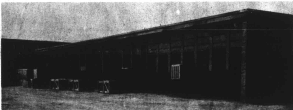
Remodeling Underway At Kelley
