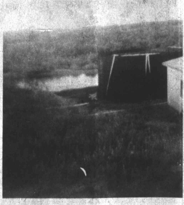
OVERFLOWING and leaking disposal holding tanks allow the pollutants to flow directly into the river.
