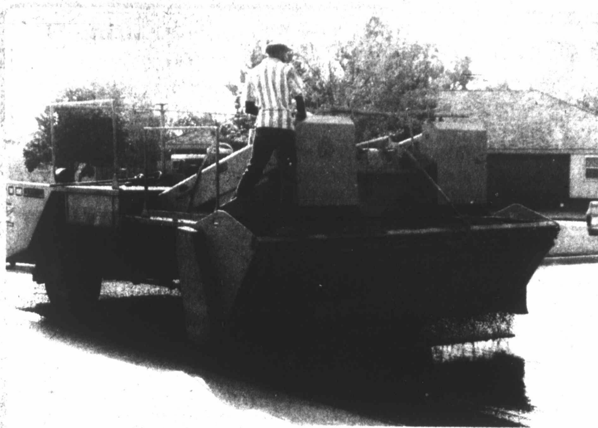
NEW COAT: Work on the seal coating operations - such as the work being shown at 17th Street - on the major thoroughfares is nearing completion, city officials report.
