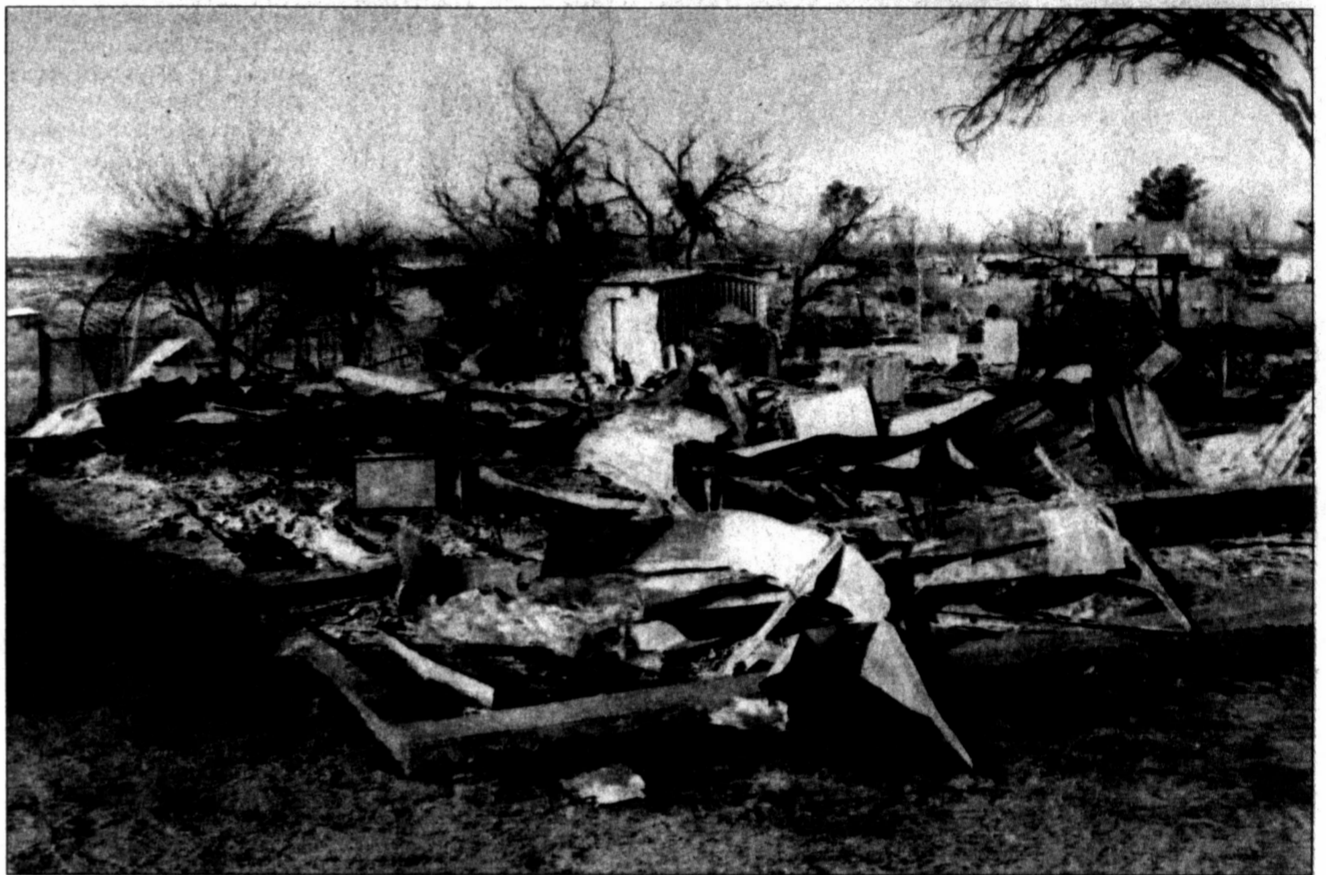
TOTAL LOSS - The home of Vicki Spray was destroyed by fire last week. The family, including Vicki and her 50-year-old son, T.J. and her adopted five-year old, lost everything. All three fire departments in the county responded to the fire that also burned two other houses and a storage shed.
