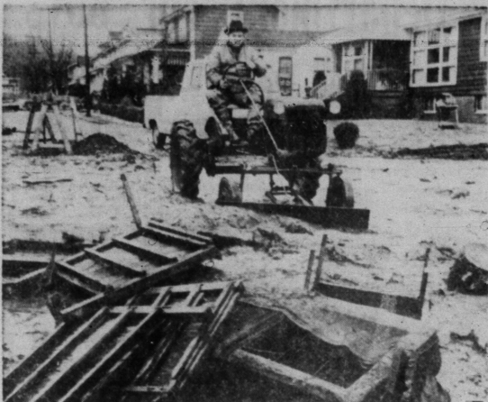
FLOOD CLEAN UP—Ed Tolbert uses a tractor to clean mud and debris from his home site in Wheeling, W. Va., which was flooded by rising waters from the Big Wheeling Creek. The cleanup was started while residents of the city kept a close watch on the rising Ohio River. (AP Wirephoto)
