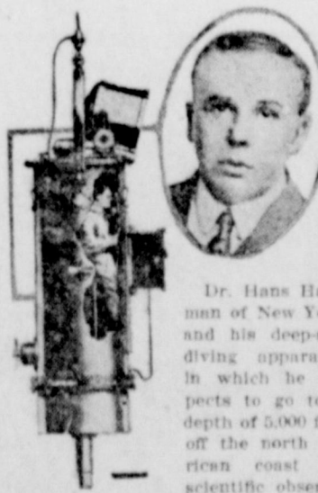
Dr. Hans Hartman of New York, who is developing a deep-sea diving apparatus in which he expects to go to a depth of 5,000 feet off the north African coast for scientific observations. He will make photographs with the camera on the front of the cylinder. Doctor Hartman is the only man to have attained a depth of 1,500 feet.
