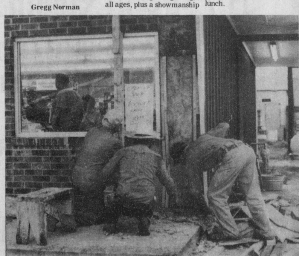
REPAIRS to the corner Kwik Korner Grocery in Bogata were being done last Friday, after the brakes failed on a 1972 Chevrolet which was driven by Stephen Wayne
