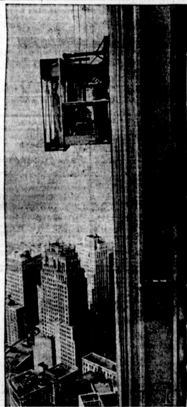
SUSPENDED WASHDAYS—With maximum safety, and still some danger involved, a window-washer stands precariously on this modern elevator-type window-washing device. Above the avenues of New York City on this 60-story building, it will take a month to wash 8,800 windows. With poor weather it may take longer. The machine is electrically operated and has a building-to-ground two-way radio for communications.
