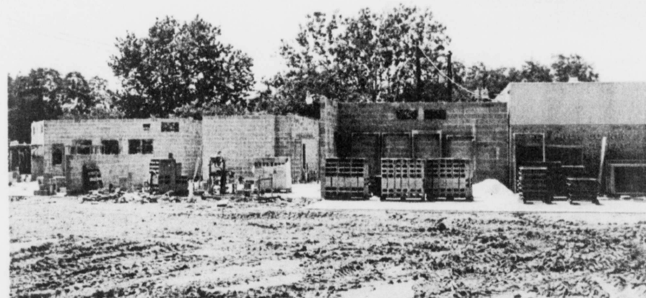
GOING UP!! Walls are going up on the new expansion of the Red River County Jail. Sheriff Bob
