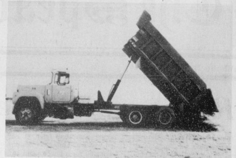
The first load of dirt for the new Spearman First National Bank was dumped at 9 a.m. Monday, July 23rd. The new bank is located at South Hwy. 207.
