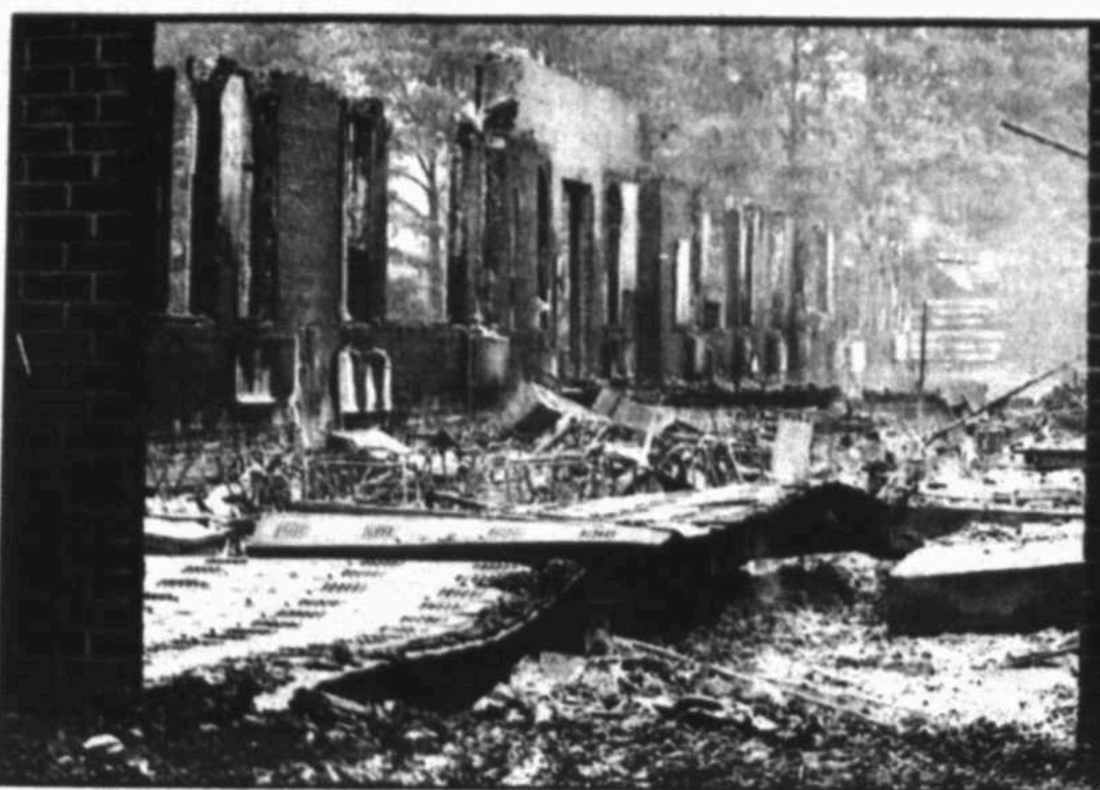
Randolph County High School in Wedowee, Ala., shown Sunday, was destroyed early Saturday morning by a fire whose cause is still under investigation.
