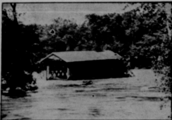
The famous old covered bridge at Housick, N. Y., pictured here, stood firm as the flood waters of the Hudson river swept around it. Nearly a concrete span, built recently to replace the old wooden covered bridge, was swept away.
