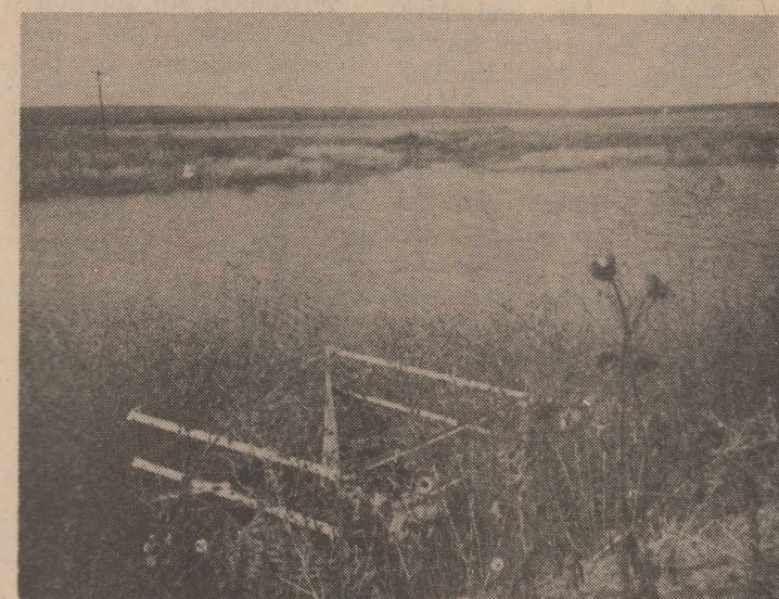
Grade Stabilization Structure
