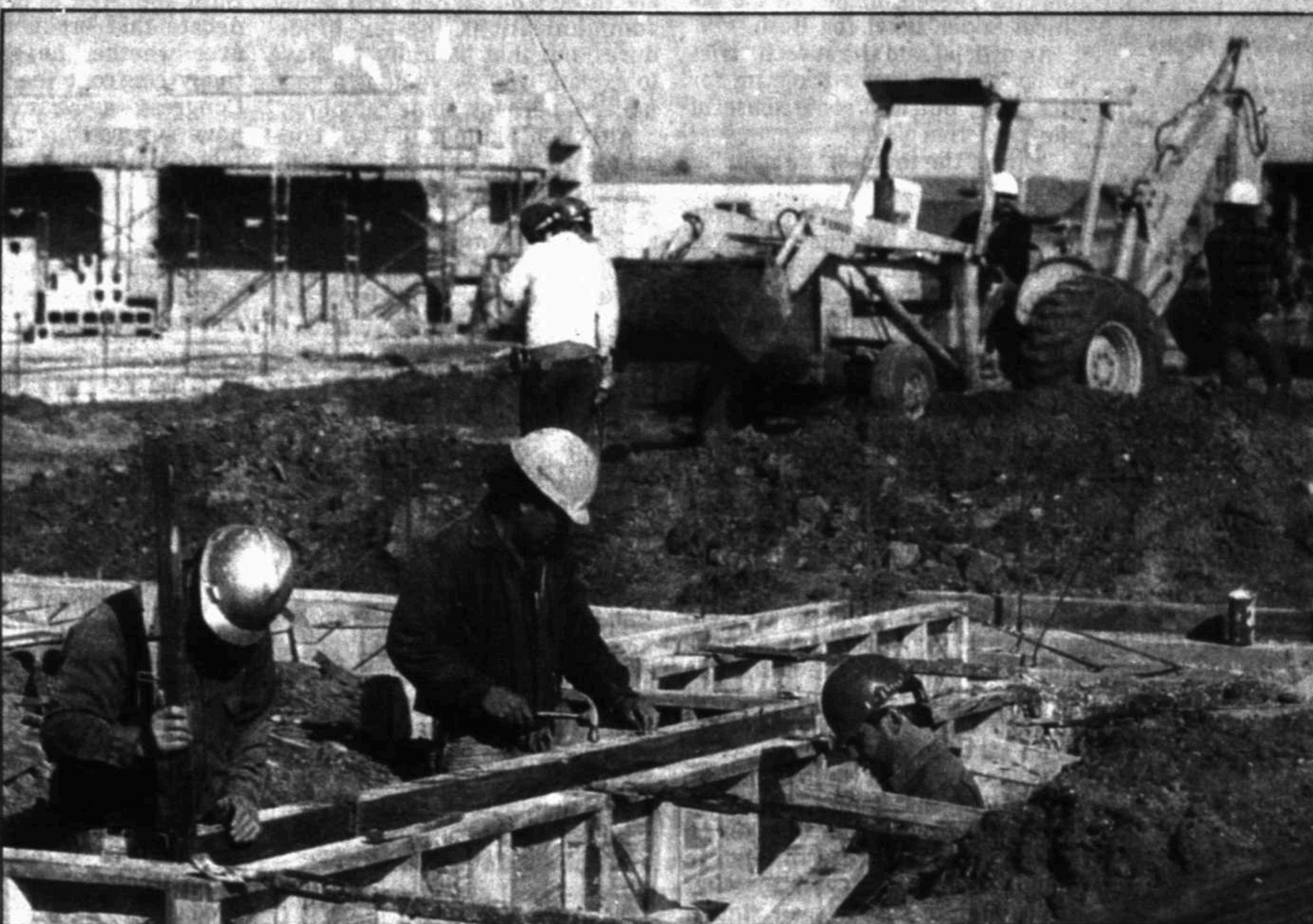
Ramon Carrasco, from left, Raymond Rosales and Keith Lewis work on Bush Elementary expansion.
