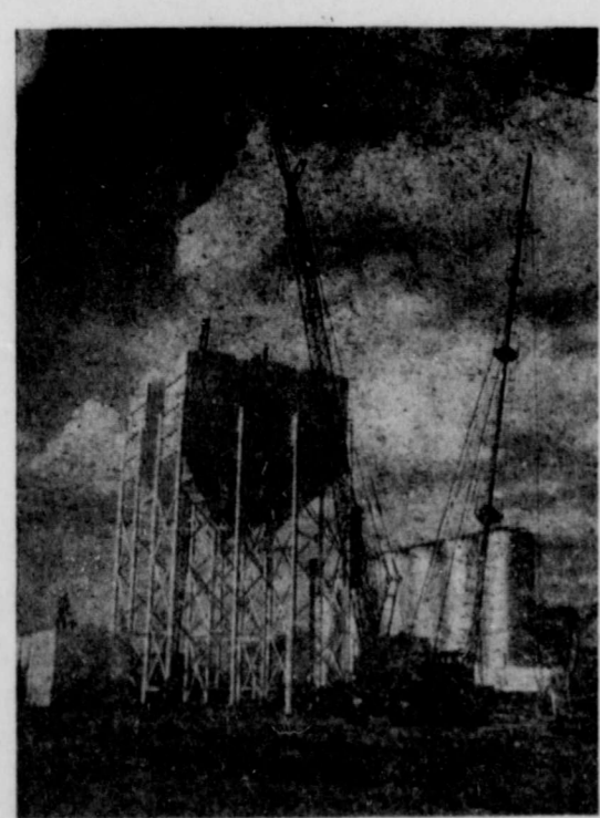
The structure shown above is part of a complex of elevated bins that will be part of the Rowland-Gordon plant being
