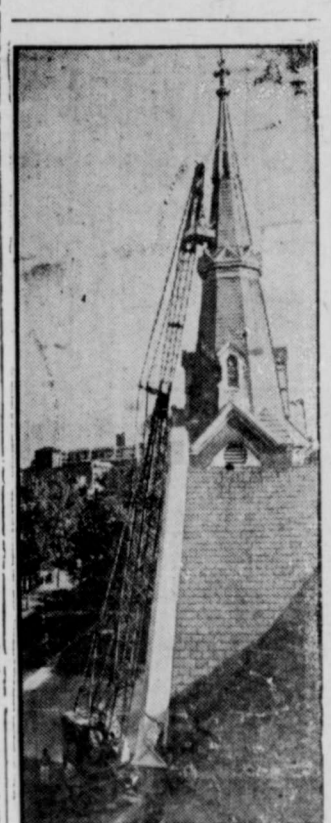
SHINGLE SHIFTER —All up in the air over his work is Jackson Davis, of Arlington, Va. Above, he repairs loose shingles on the steeple of a Washington, D.C., church. Davis, an employee of a roofing and sheetmetal company, is suspended in a wooden basket seat from a huge crane.
