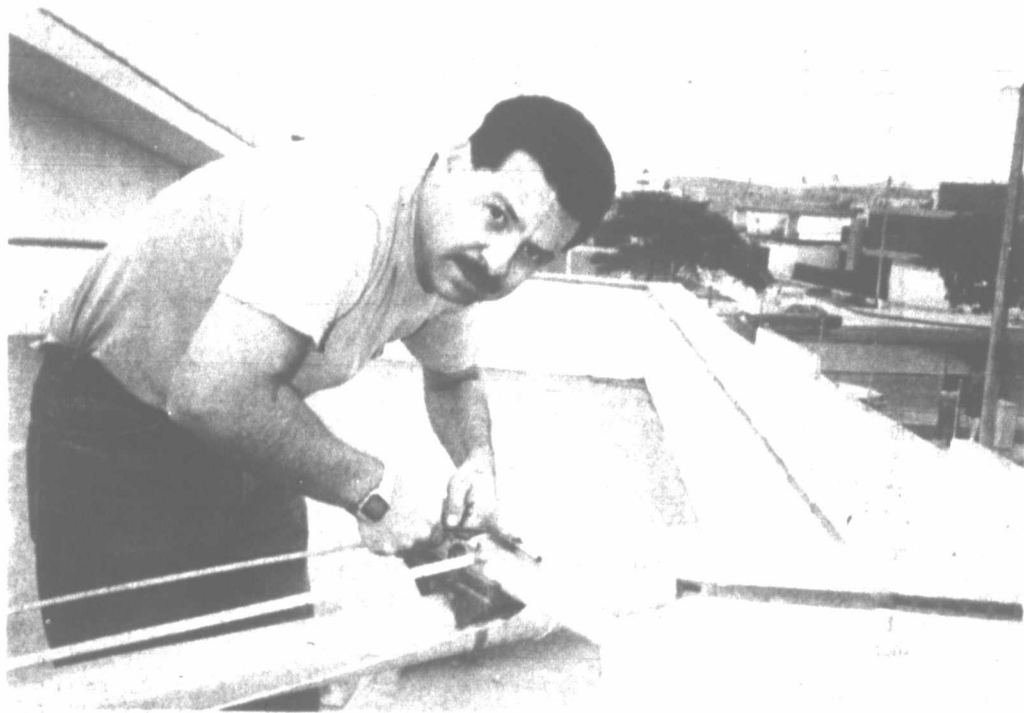
MSgt. George D. Rivera performs corrosion control on a Mission Radio System or MRS antenna on top of the Military Aid and Assistance Group building in Lima, Peru. Rivera was one of a four-man team from the 1978th Information Systems Group here who recently performed an annual maintenance visit to Peru, in support of the MRS.
