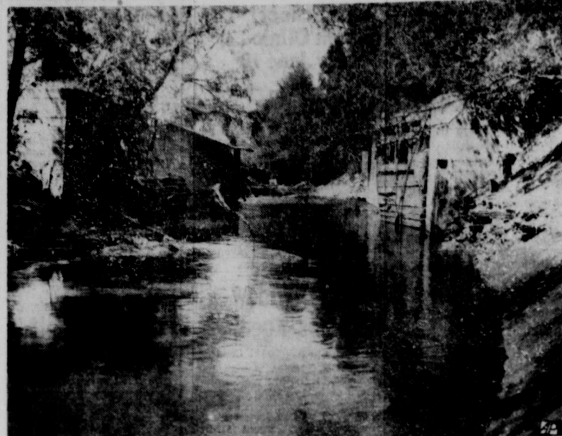
DALLAS STEAMBOAT LOCKS —These are part of the old steamboat locks and dam built forty-four years ago when Dallas had dreams of being a riverboat town. The locks are on the Dr. James J. Hammett place a mile down the Trinity River from the Dallas city limits. The concrete is about to fall out of the flood gates and the gates are loose on their hinges. The locks are submerged when the river is a flood. (UPI Photo)
