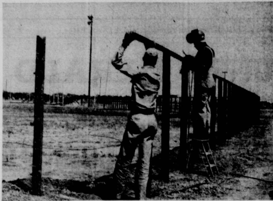
FENCE FOR BALL PARK—Kermit Johnson, left, and Bob Steen, with the welder helmet, are shown putting up a section of the new steel fence at the fair grounds ball diamond. The fence is all metal, with the posts set in concrete. With the erection of a large steel backstop, building of this fence, and the completion of permanent steel bleachers, the Perryton ball field will be one of the best in the Panhandle.
