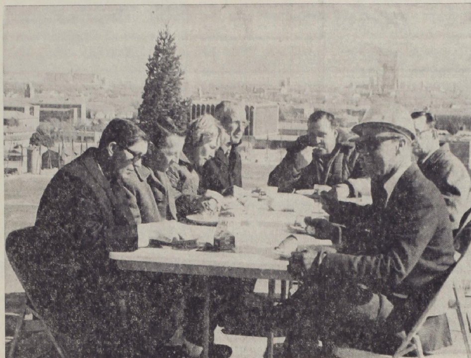
ROOFTOP LUNCHEON HELD—Eating lunch atop the newly completed first section of the roof slab for Weymouth Hall in the Wiggins Complex Wednesday were some of the people instrumental in the project. Seated around the table from left are Howard Schmidt, project
