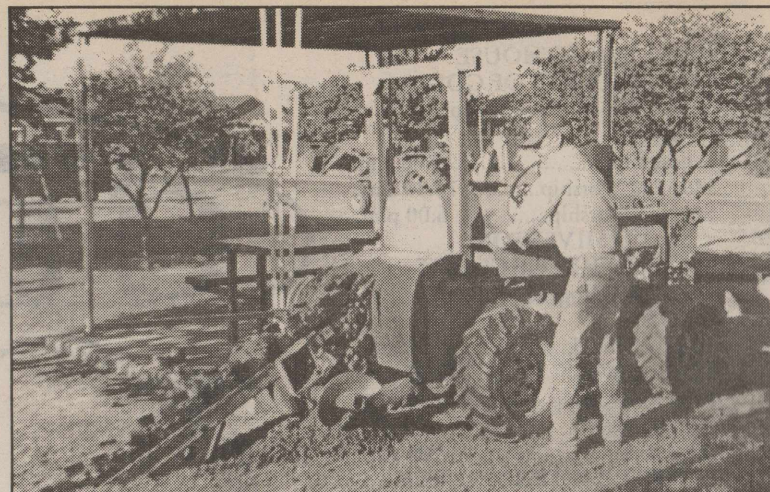
City Water Superintendent Thomas Lee Perkins has been installing an underground sprinkler irrigation system for watering the Silverton City Park. Watering will be done automatically at night, and this should help keep the park green during drier years as well as saving the City money on the expense of watering. Briscoe County News Photo
