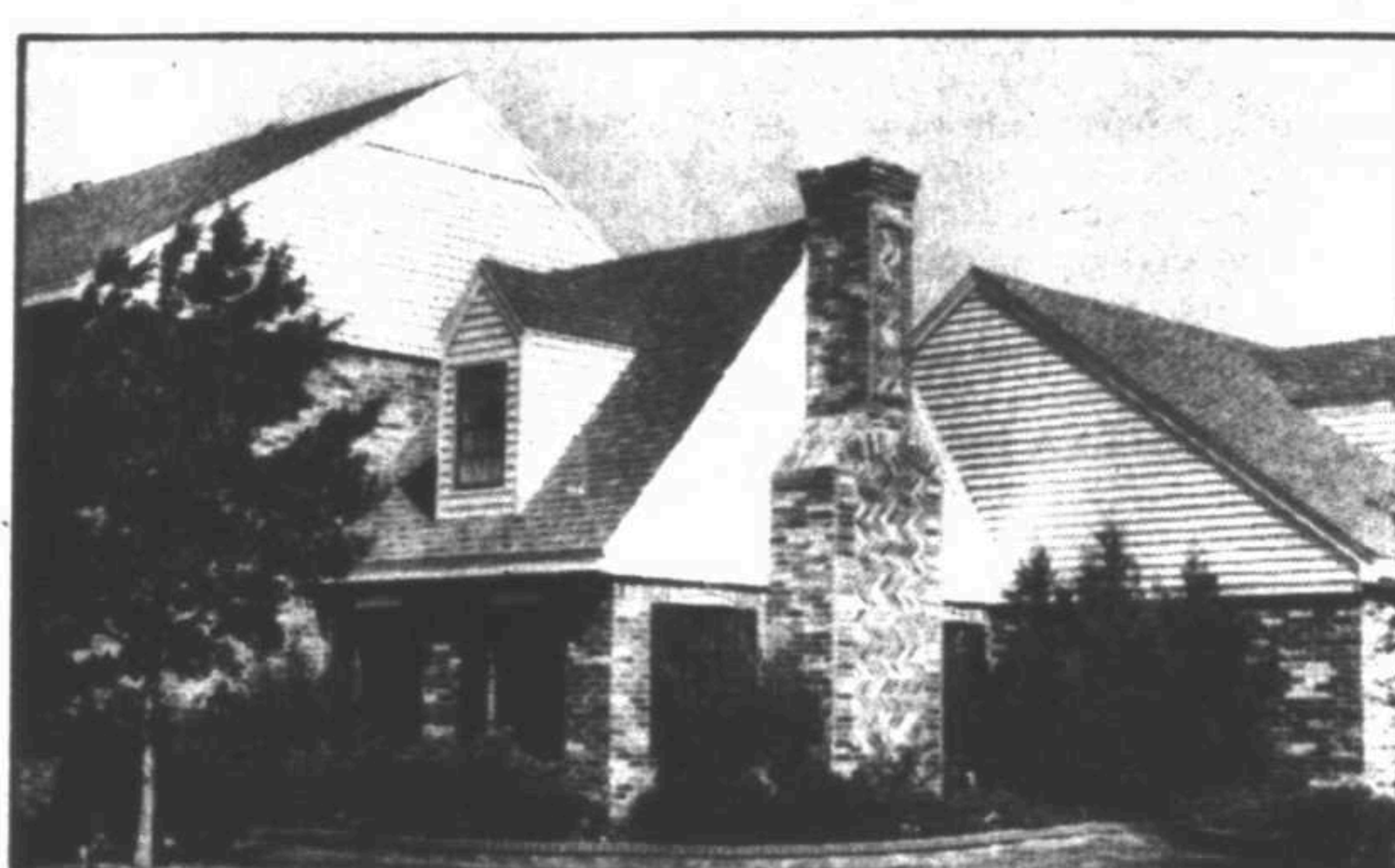
This beautiful home in the Green Tree subdivision is enhanced by the addition of vinyl siding and custom shutters by Lewellen Construction Company.
