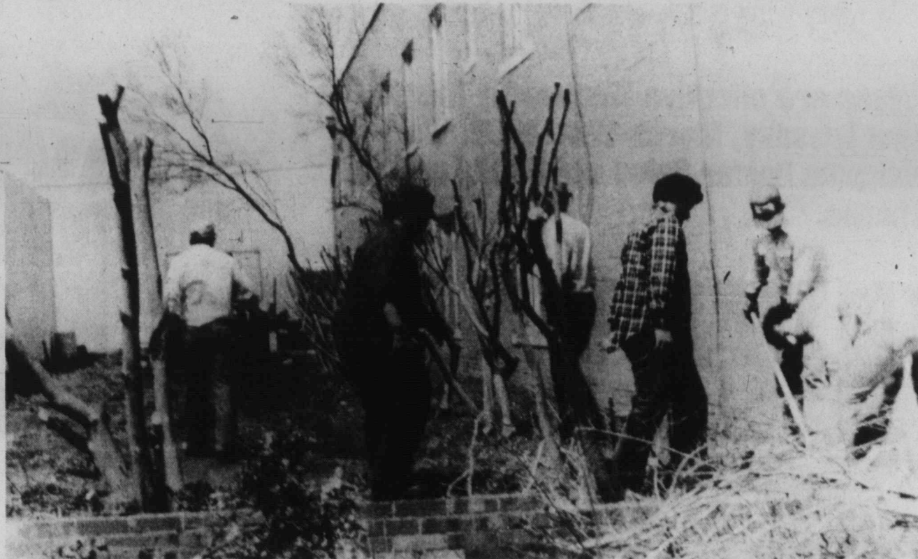
CLEAN-UP VOLUNTEERS — Chamber of Commerce directors volunteered to help Chamberettes in the renovation project of the Keltner Hotel by cleaning up the vacant lot next to the building, in the spring of 1983. The men chopped weeds, bushes and debris in the lot that had been deteriorating for years.
