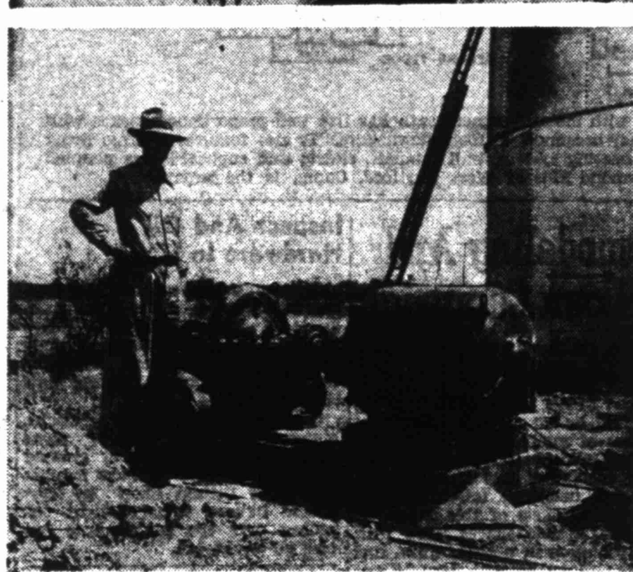
Picture No. 1—Twenty-inch transit pipe for the 9,000-foot water line is strung out along line's right-of-way. No. 2—The huge ditch-digging machine is providing a ditch 36 inches wide and six feet in depth. No. 3—A section of the pipe is being put in place by a pipe crew which follows the ditch-digging machine. No. 4—Henry Nunn, city water superintendent, inspects the new booster pump which recently was installed at the Wadley tract.
