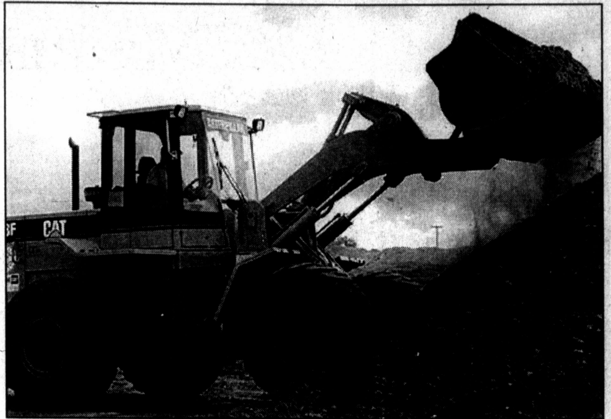
DIRT WORK is well underway on 23 acres at Rogers Road and South Interstate 20 where construction on Mitchell County's new hospital and physicians' clinic is scheduled to begin. County road and bridge crews are preparing for the contractor's arrival.
