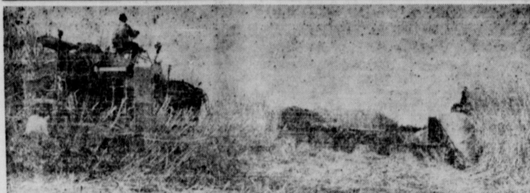
The days when hundreds of laborers used to cut the sugar cane by hand and mules slowly pulled the wagons to the sugar mill, are gone. Today Thomson "Hurricane" harvesters cut, top and stalk a hundred tons of cane a day and specially designed Allis-Chalmers cane tractors speed two or three heaped cane wagons at a time to the mill.
